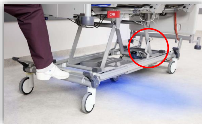
IndiGo cabling - location
