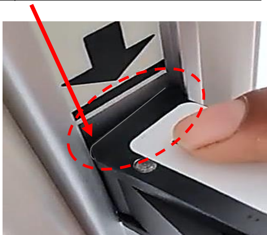
Fig 3 Incorrect installation due to defective dovetail mount accessory (gap or opening presence)
