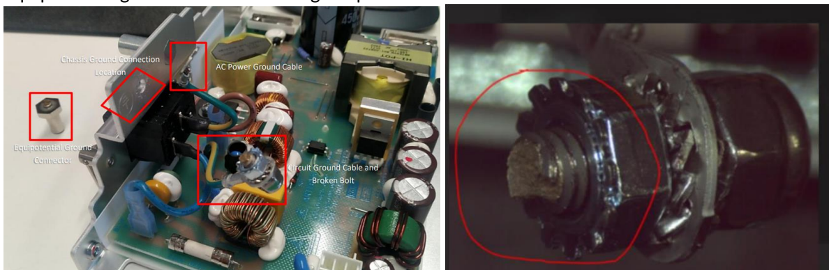
Figure 1. Power Supply Chassis and Circuit with Disconnected Ground Wires and Broken Ground Bolt
